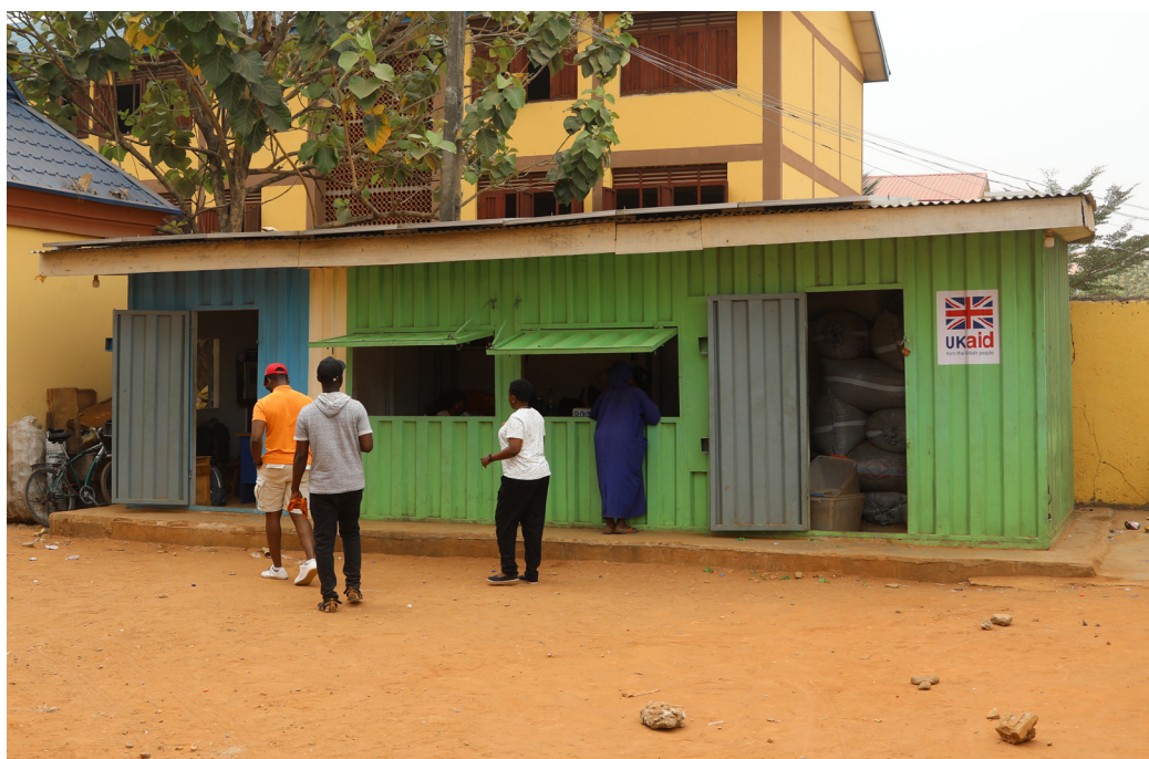
← Image 6. GIVO-Warwick collection centre equipped with solar roof panels. The centre serves as a decentralized hub for the collection, aggregation and digital tracking of plastic waste.
