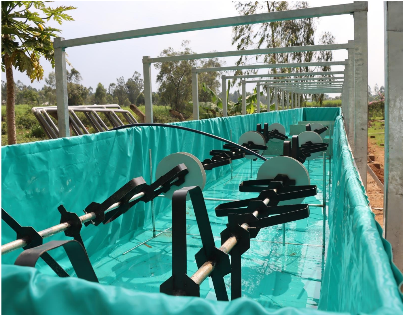
Photo 8: Biogas Plant construction at RioFish Limited, Opapo Market
